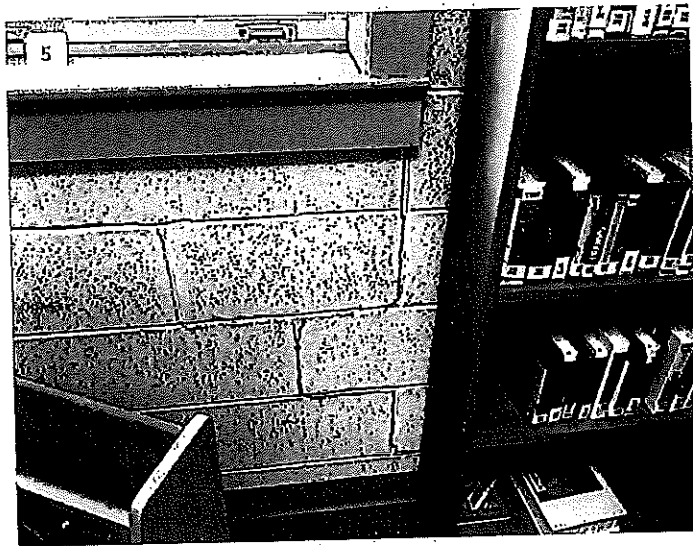
a.5: Height of Cracking Extending to Concrete Slab
