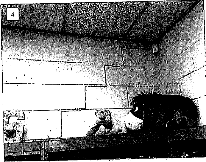
a.4: Cracking in Northwest Corner of Wall
