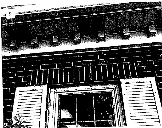
b.1: Exterior Cracking Above Window
